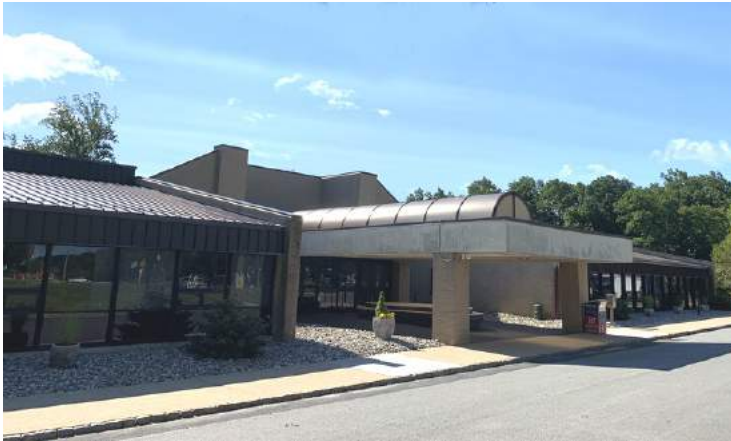
Municipal Building, 502 Millbrook Ave, Randolph, NJ 07869
